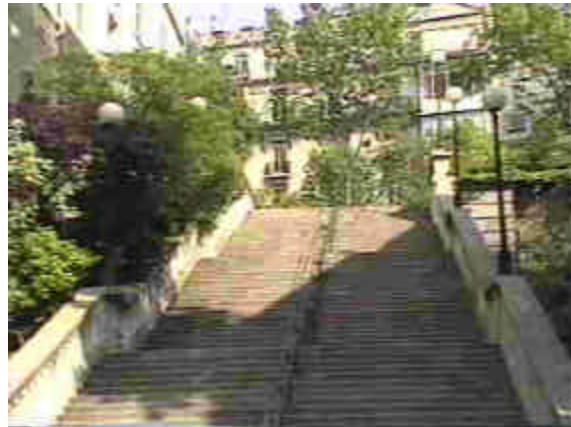
Looking up a step street leading from the Debilly Footbridge to Avenue President Wilson.
